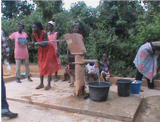
A working pump after the repair
