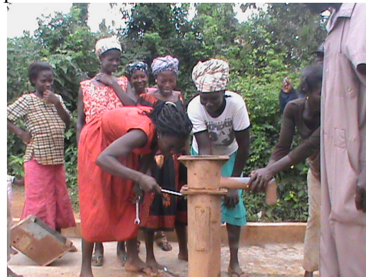
Working on a broken pump
