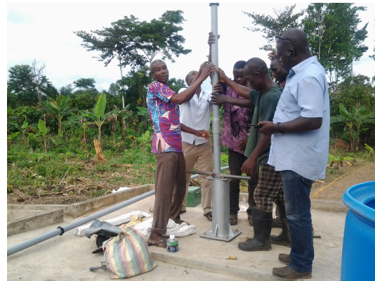
Installing pipe for the new pump
