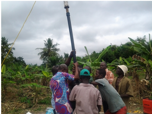
Broken pipe being lifted
