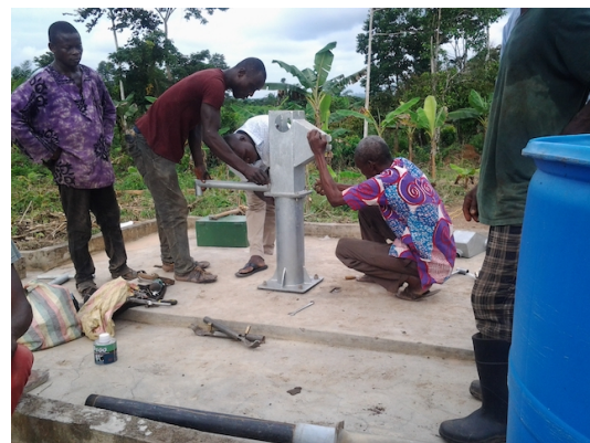
Assembling the new pump
