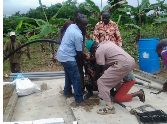
Old flexible pipe being removed
