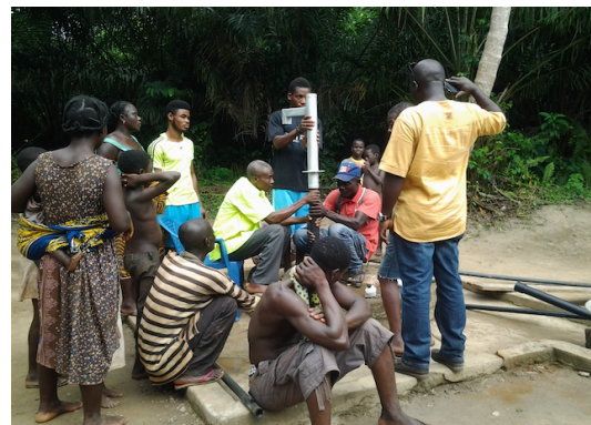
Pump repair in progress.
