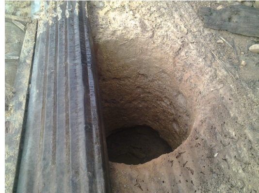
Start of a family latrine
