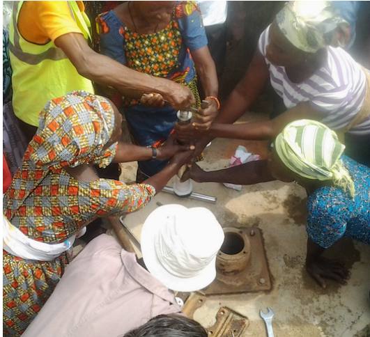
Repairing a broken pump
